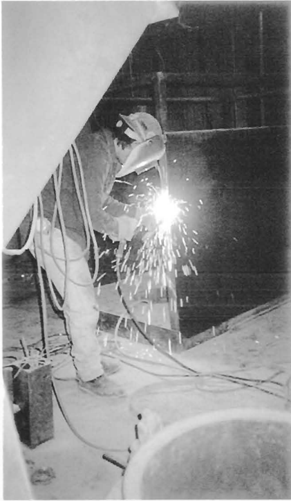
On-site fabrication assembly was carried out on the precipitator after an 18-week dismantling process revealed extra damage caused by the fire.
