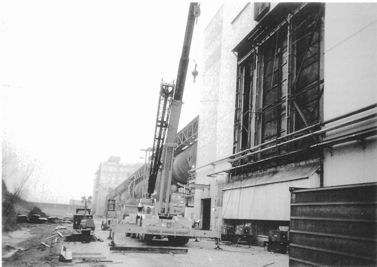
New collecting plates are being installed in the lower precipitator at Holnam Cement's Clarksville, Missouri, U.S.A., plant.
